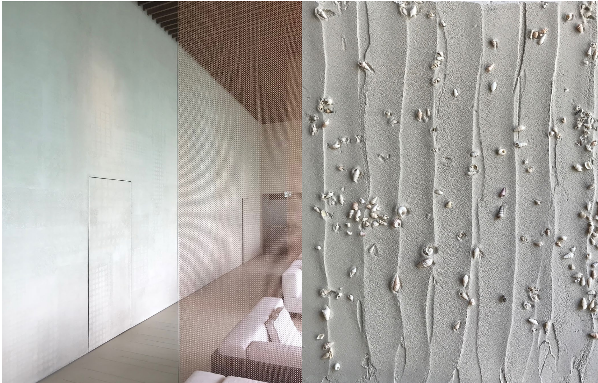
TerraEvoca 2 layers with a custom color (left) obtained mixing ground local seashells with clay (right), Katara Restaurant, Doha, Qatar
